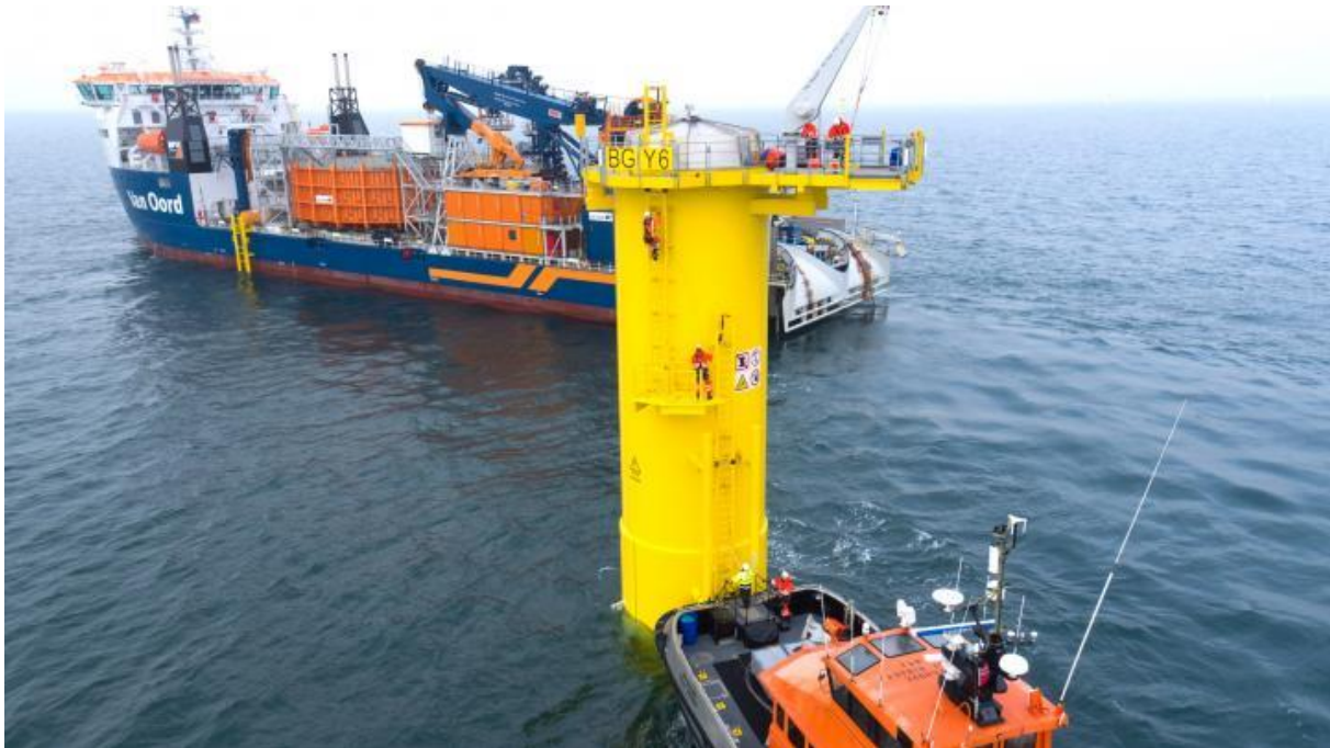
Figure 28: Van Oord's Nexus Cablesip installing cable at a wind turbine monopile
