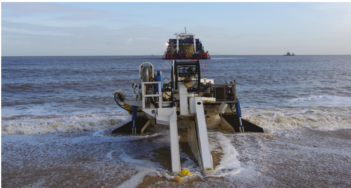
Figure 20: Enshore Subsea's PCP-2 cable plough
